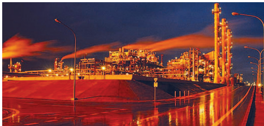
An oil refinery in Mina-Al-Ahmadi, Kuwait.
