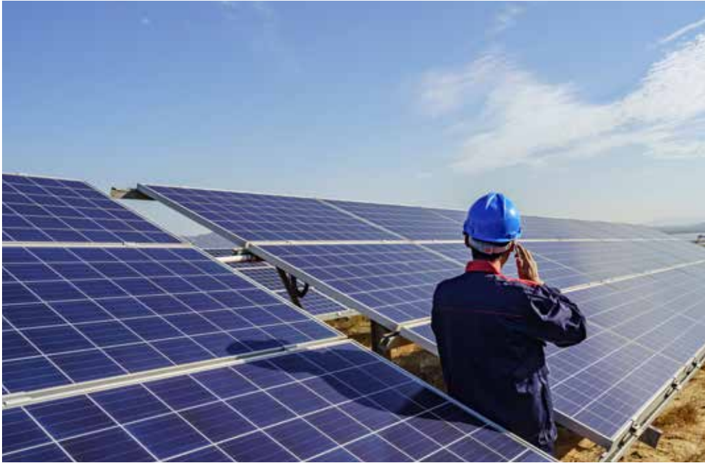
An engineer checks solar panels in China. Since 2015, China has been the largest producer and buyer of solar panels. It is number two in producing the most solar energy, just behind Germany and ahead of Japan, Italy, and the United States.
